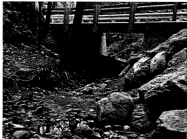
Abutment and bridge design on site with complicated and diverse subgrade, mixture of soil and bedrock – Looking downstream.
